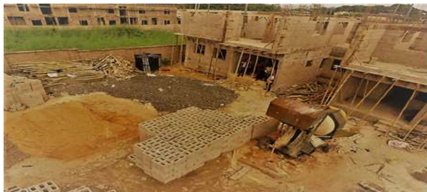
Figure 8. Aerial reality image of material and equipment onsite during closing hour including offcuts scattered on the floor. captured by a DJI Phantom 3 Standard drone. Source: Field survey 2019.
