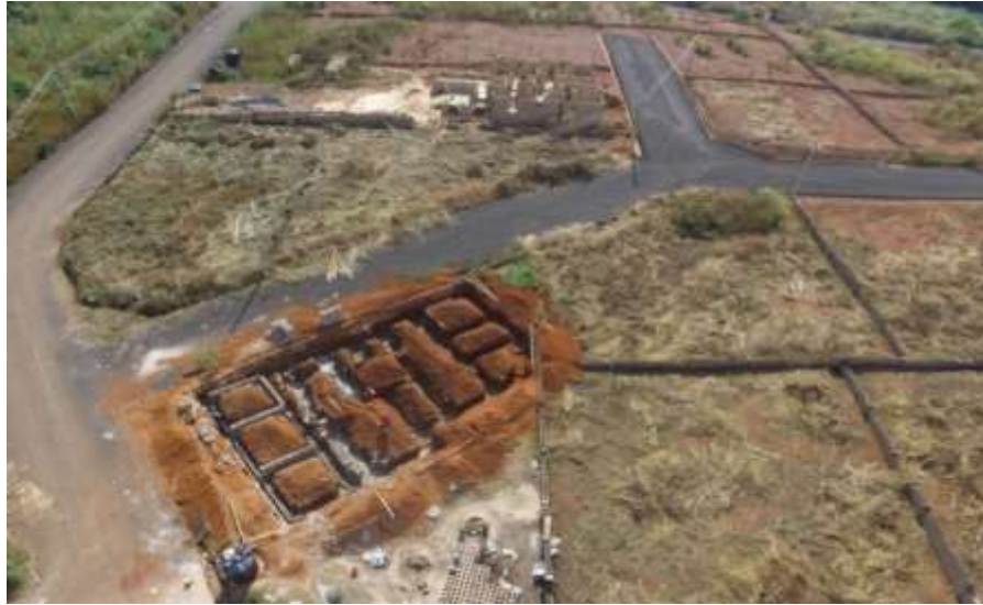
Figure 4. Aerial view of devine hectares estate. Source: Field survey 2019.
